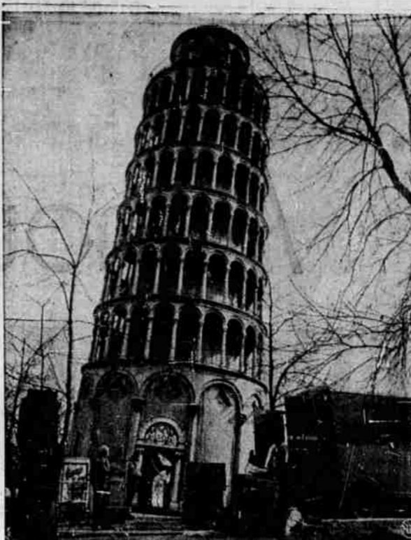
"PLUMB TIRED" OF LEANING—Robert A. Ilg, Chicago manufacturer, bids goodbye to his old home, which is a replica of Italy's famed leaning tower of Pisa. Ilg is moving to California, where he hopes to be able to live on the level.
