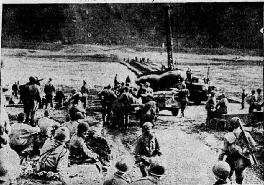
Third Army engineers lay down a pontoon bridge across the Moselle river in a dress rehearsal for crossing of the Rhine, which was made in conjunction with a crossing by three other armies in a final push against Germany. Scenes like this were duplicated for miles up the broad stream.
