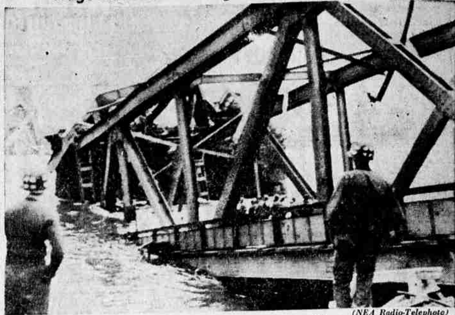
First Army medical corpsmen stand by ready to aid comrades being rescued from wreckage of collapsed center span of 1200-foot Ludendorff Bridge at Remagen, which served as first span to funnel Yanks across the Rhine River. The bridge collapsed while undergoing repairs, plunging hundreds of men into the river, but engineers report the vital span will soon be in operation. Signal Corps photo.
