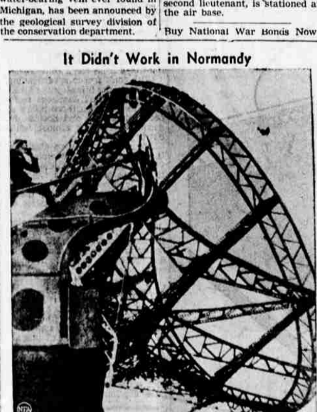
Germans say this huge gadget is an aircraft detector which sends out great magnetic waves which warn of approach of Allied planes. Nazi caption on photo, obtained through neutral source, did not mention whether any of the gadgets had been operating in Normandy on D-Day.
