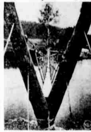
Engineer battalion at Ft. Leonard Wood, Mo., built this cable-supported toggle bridge in a matter of minutes. "V" shape is practical as well as symbolic. (Signal Corps photo.)
