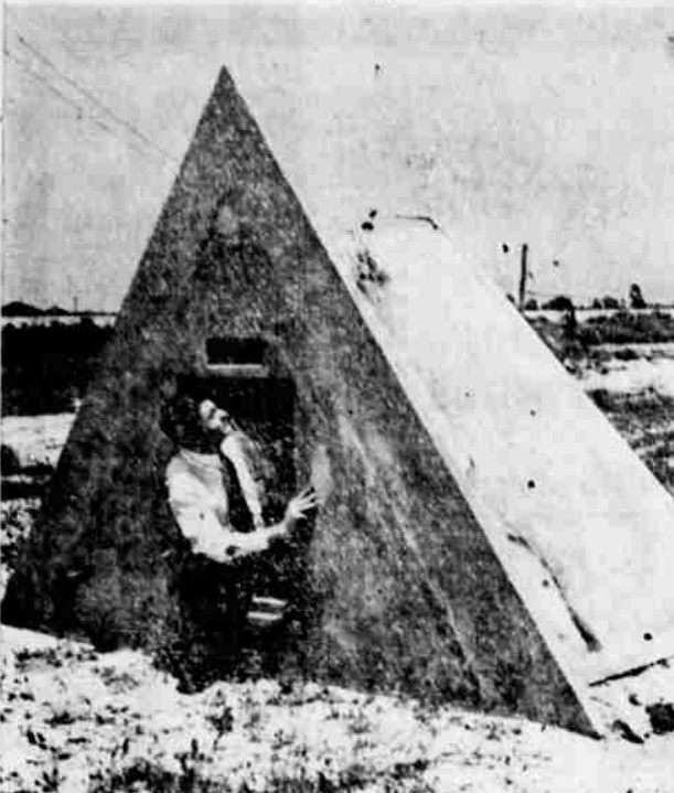
The West Coast's first commercially produced air raid shelter is this steeply pitched concrete affair being produced by a North Hollywood, Calif., concern. It sells for about $100, goes up in 48 hours and can readily be adapted for mass production.
