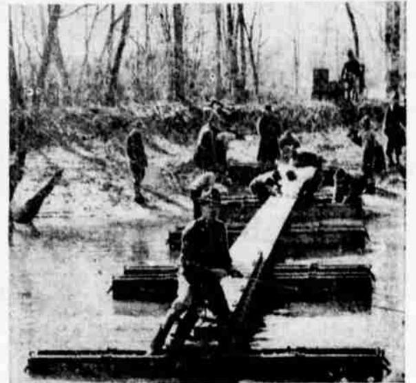
ENGINEERS BRUSH UP—Units of 121st Engineers construct 72-foot pontoon bridge across Patuxent River at Fort Meade, Md., as part of their training under defense program.
