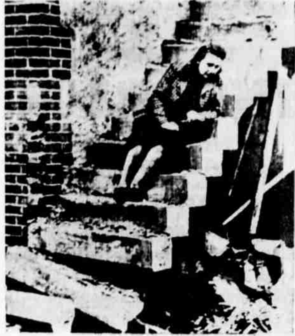
(NEA Cable-Telephoto) Surveying wreckage of what was once her home, a young London suburbanite sits on steps and wonders what to do about the damage done to it by Hitler's "airblitz" of Aug. 16. She kept safe during the raid in an air shelter. Picture and caption passed by British censor, picture cabled to New York.
