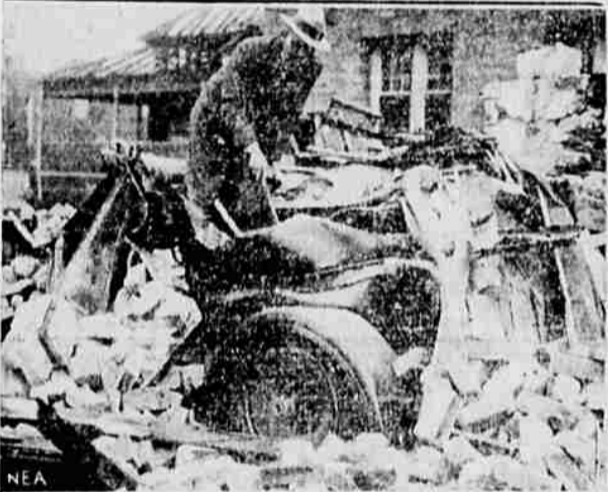
Here is the danger that threatened pedestrians. This car was completely wrecked by falling bricks at Long Beach.
