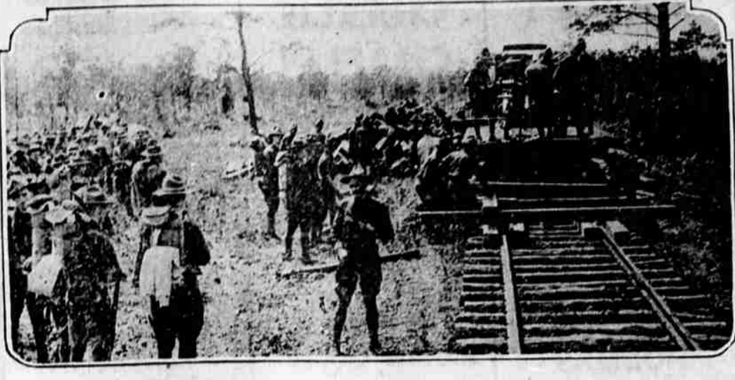
Photo by American Press Association. Guardsmen quickly pick up the business of railroad construction. At a camp "somewhere on Long Island, New York," guardsmen are shown laying ties of a railroad on which food will be brought to the camp.
