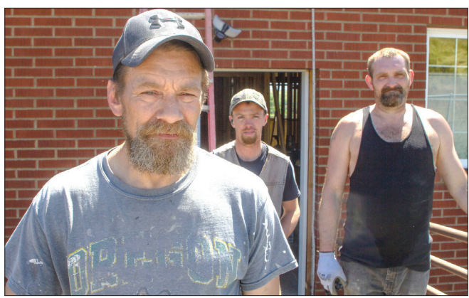
Yasser Marte/East Oregonian From left, construction workers Leon Sauers, Terry Johnson and Joe Tenbusch work Tuesday, June 21, 2022, to convert the former U.S. Forest Service building at 2601 S.W. Hailey Ave., Pendleton, into an apartment complex.
