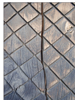
Bennett Hall/Blue Mountain Eagle The totem pole's unprotected wood has been badly weathered by the elements.
