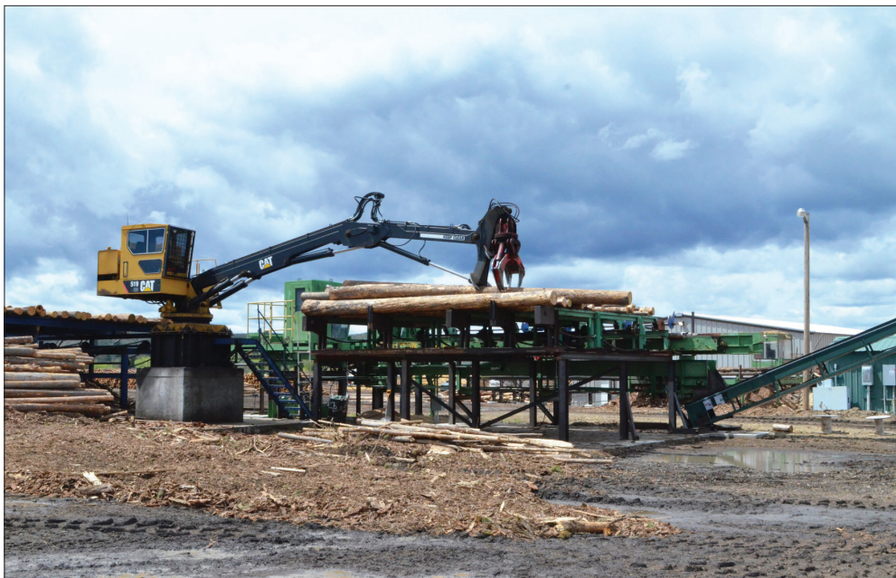
Richard Hanners/Blue Mountain Eagle, File Raw logs ready to be milled at Iron Triangle's post and pole plant in Seneca. The plant is one example of investments made by the company to carry out its 10-year stewardship contract with the Malheur National Forest.
