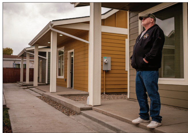
Alex Wittwer/EO Media Group, File Dennis Scudder, an Army veteran, looks over his new neighborhood in La Grande on Nov. 4, 2021. Scudder bounced between temporary housing solutions before moving into Veteran Village Union County, a new community of cottage-style homes.
