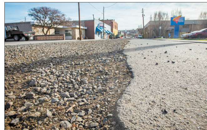
Ben Lonergan/East Oregonian Gravel fills a utility cut along Southeast Second Street near Southeast Byers Avenue on Thursday, Dec. 2, 2021, in downtown Pendleton.
