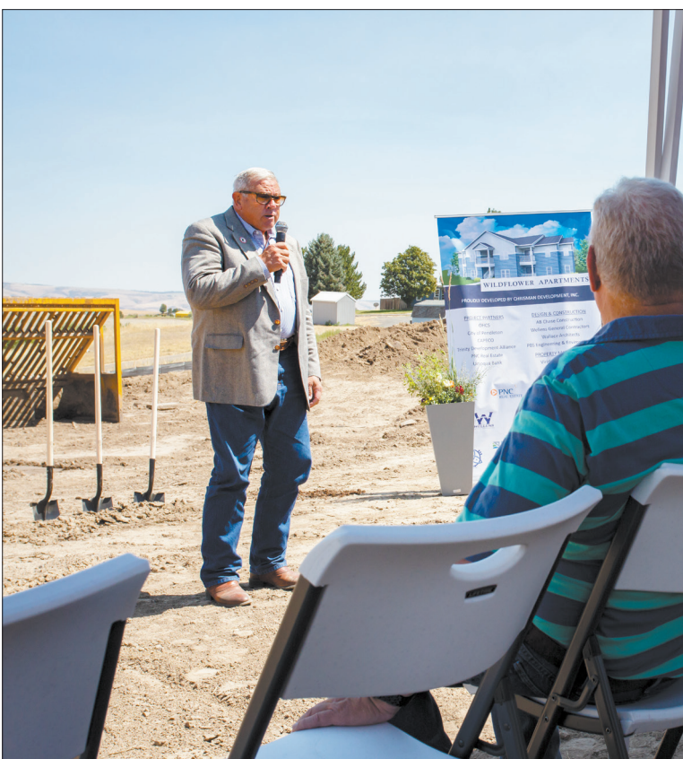
Pendleton Mayor John Turner speaks Wednesday, July 21, 2021, during a groundbreaking for the new Wildflower Apartments, an 80-unit affordable housing development on Southwest 18th Street in Pendleton.
