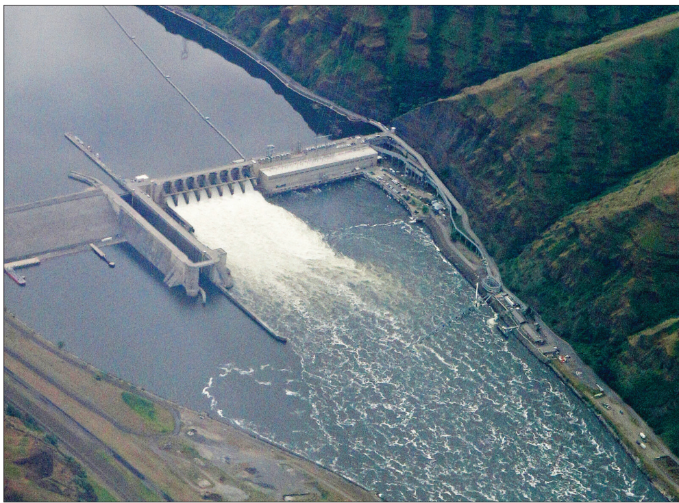
The Lower Granite Dam on the Snake River is seen from the air near Colfax, Washington. A Republican congressman has proposed removing four hydroelectric dams in the Northwest, including the Lower Granite Dam, as part of a sweeping plan to save salmon populations and provide aid to farmers and others.
