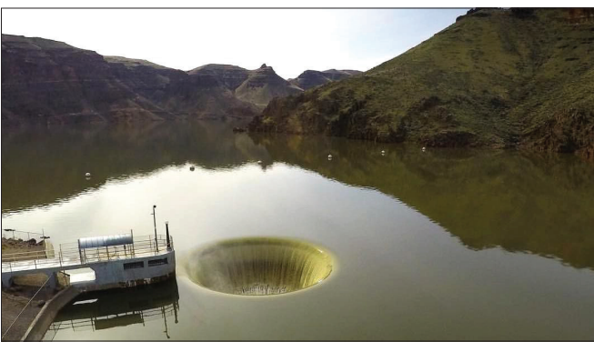
The "glory hole" at the Owyhee Reservoir funnels excess water into the spillway and into the river below the dam.
