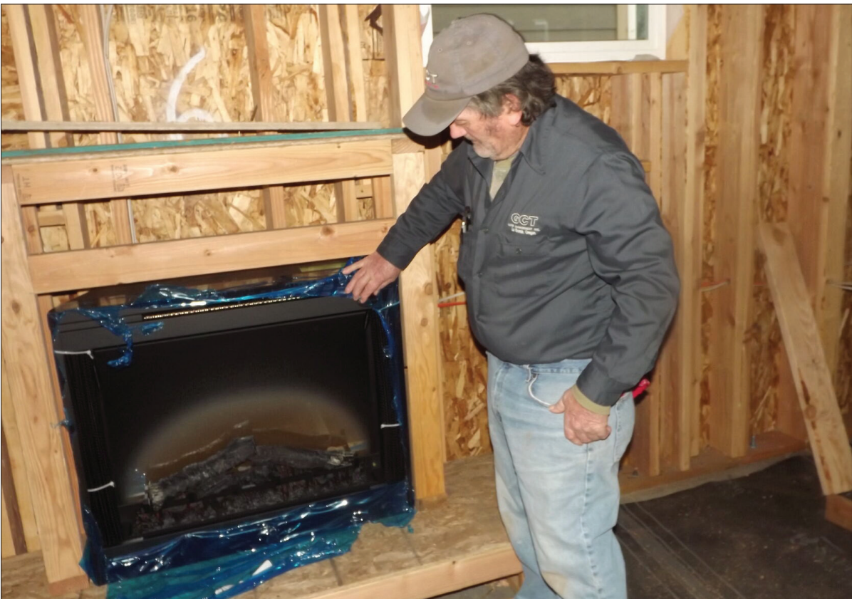
Dick Mason/The Observer/La Grande Observer Bob Haley, of GCT Land Management, examines an electric fireplace Tuesday, Dec. 15, 2020, in one of the homes under construction at Veterans Village Union County in La Grande.
