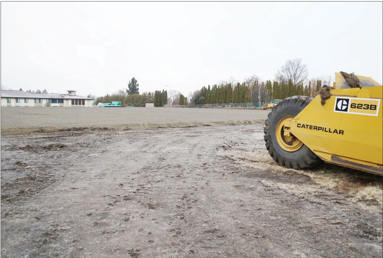
Heavy machinery sits beside a large leveled lot next door to Eastern Oregon University’s Community Stadium on Monday, Dec. 7, 2020, where work is underway to build a new fieldhouse that will supplement the university’s sporting programs.
