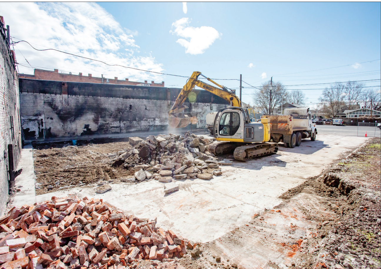
An excavator removes rubble from the site of the former We Sell Stuff building at 342 S.W. First St. in Pendleton on Tuesday afternoon. The building, which was severely damaged in a fire on Sept. 29, 2019, was torn down over the course of the last several weeks.
