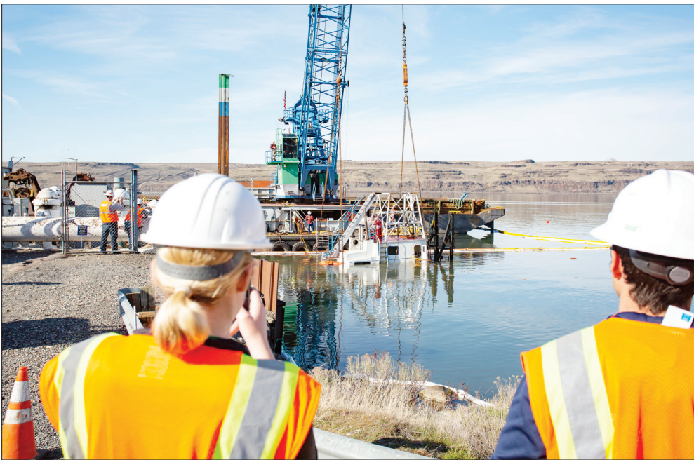
Representatives from various environmental agencies watch as the Tug Nova, a 38-foot tugboat owned by HME Construction, is raised from the Columbia River 10 miles north of Umatilla on Thursday afternoon.
