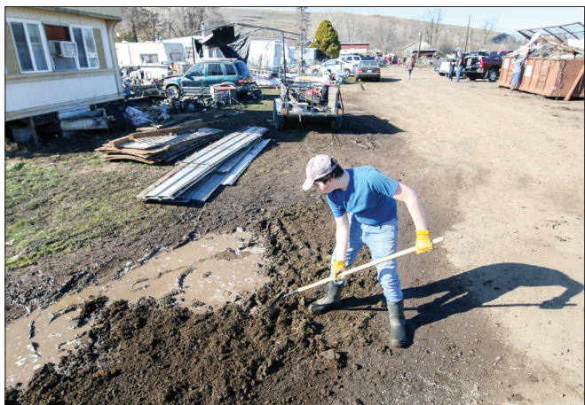
Staff photo by Kathy Aney Nathan Burcham, 14, shovels dirt into a puddle on Saturday as part of the church's effort to clean up flood damage at Hall's Trailer Park.
