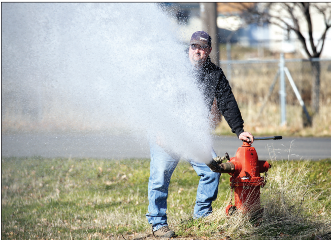
Staff photo by Kathy Aney Athena Public Works Manager Ken Faircloth flushes a hydrant on Friday as the city worked to clear its water system of coliform bacteria.
