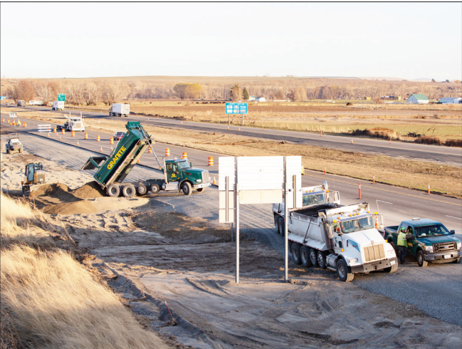
Crews work to repair the shoulder of Interstate 84 near Milepost 187 outside of Stanfield on Wednesday afternoon.
