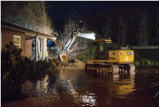
Staff photo by Ben Lonergan Pendleton Public Works crews use an excavator to pack gravel and rock into a hole in the levee behind the East Oregonian office in Pendleton.
