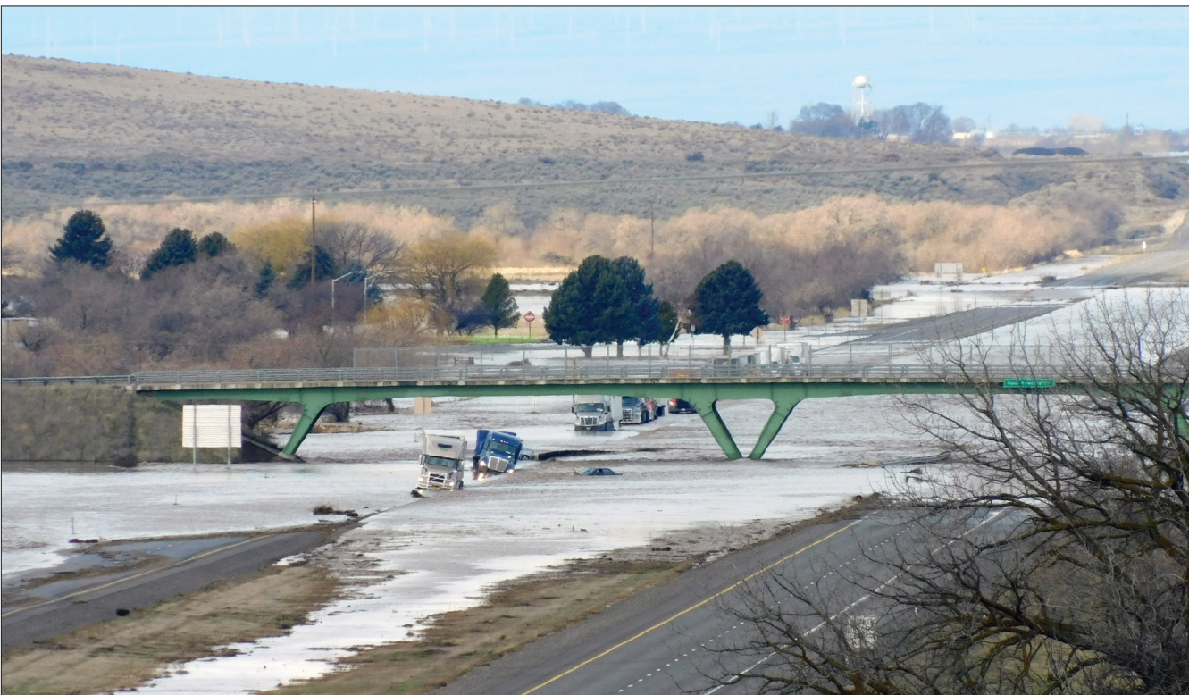
Trucks sit in flood water covering Interstate 84 just west of milepost 188 at the Pilot truck stop at Stanfield.
