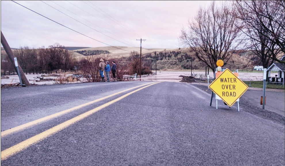
A sign warns of the floodwaters ahead on South Walla Walla River Road on Thursday evening in Milton-Freewater.
