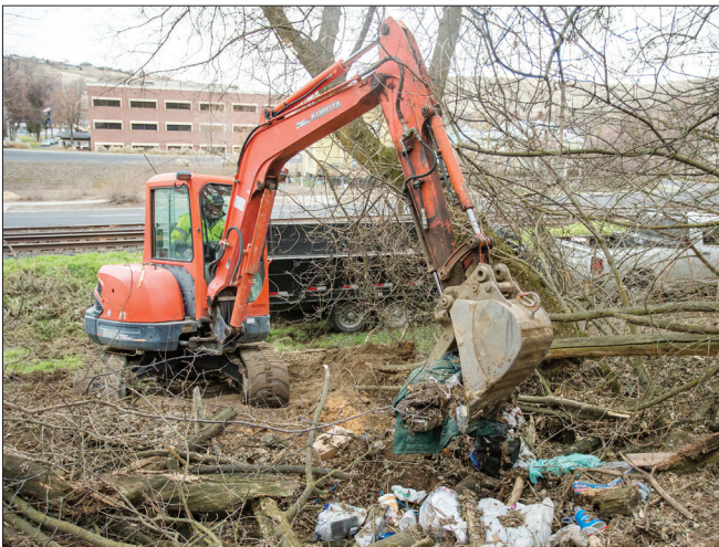
A city employee uses an excavator to clear refuse from a tract of city property near the railroad tracks at the corner of Southeast Frazer Avenue and Southeast 10th Street in Pendleton on Friday morning. The site had been used as an illicit storage site.
