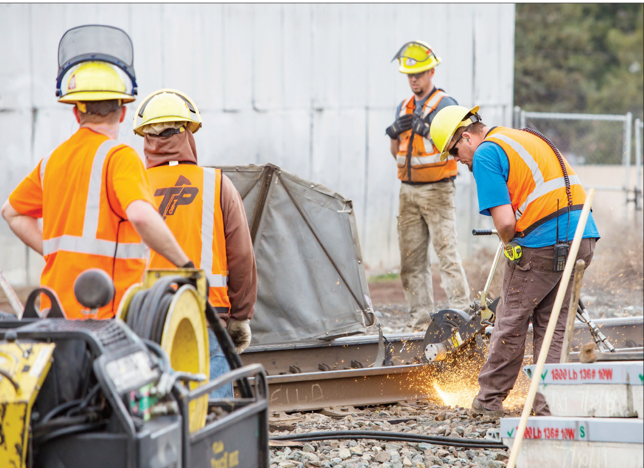
Staff photo by Ben Lonergan A railroad worker cuts a length of track while working on replacing the railroad crossing on Southeast 17th Street near Southeast Court Place on Tuesday afternoon. The replacement was a joint project between RoadSafe and Union Pacific Railroad, according to an email from city engineer Tim Simons. Workers on site said this was the first of three railroad crossing replacements in the Pendleton area.
