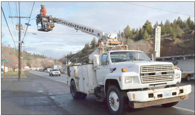
EO Media Group file photo A crew runs an optical fiber cable along South Canyon Boulevard from the John Day Fire Hall to the Grant County Education Service District building on April 3, 2019. A $6 million USDA grant announced Tuesday will provide high-speed internet access to Long Creek, Monument and Seneca.
