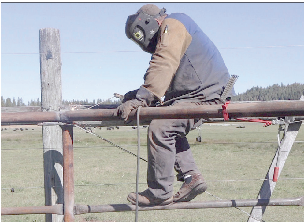
Crews finished installing a 5-foot-tall, 3-mile-long wildlife fence at Mill-Mar Ranch in southwest Oregon on Nov. 4 to keep wolves from preying on cattle.
