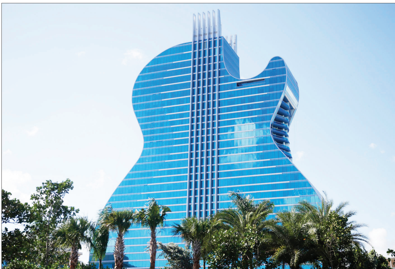
The guitar shaped hotel is seen at the Seminole Hard Rock Hotel and Casino in Hollywood, Fla. The Guitar Hotel's grand opening is on the tribe's land in Hollywood. It's the latest step in the Seminole Hard Rock empire, which includes naming rights on the Miami-area stadium where the 2020 Super Bowl will be played.
