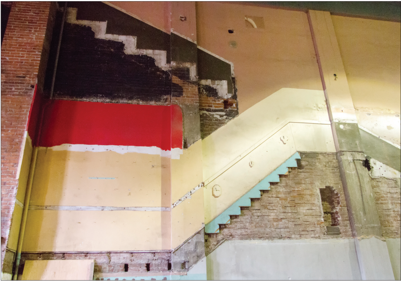
A mosaic of colors on the Rivoli’s south wall marks old stairs and a balcony removed from the historic building.
