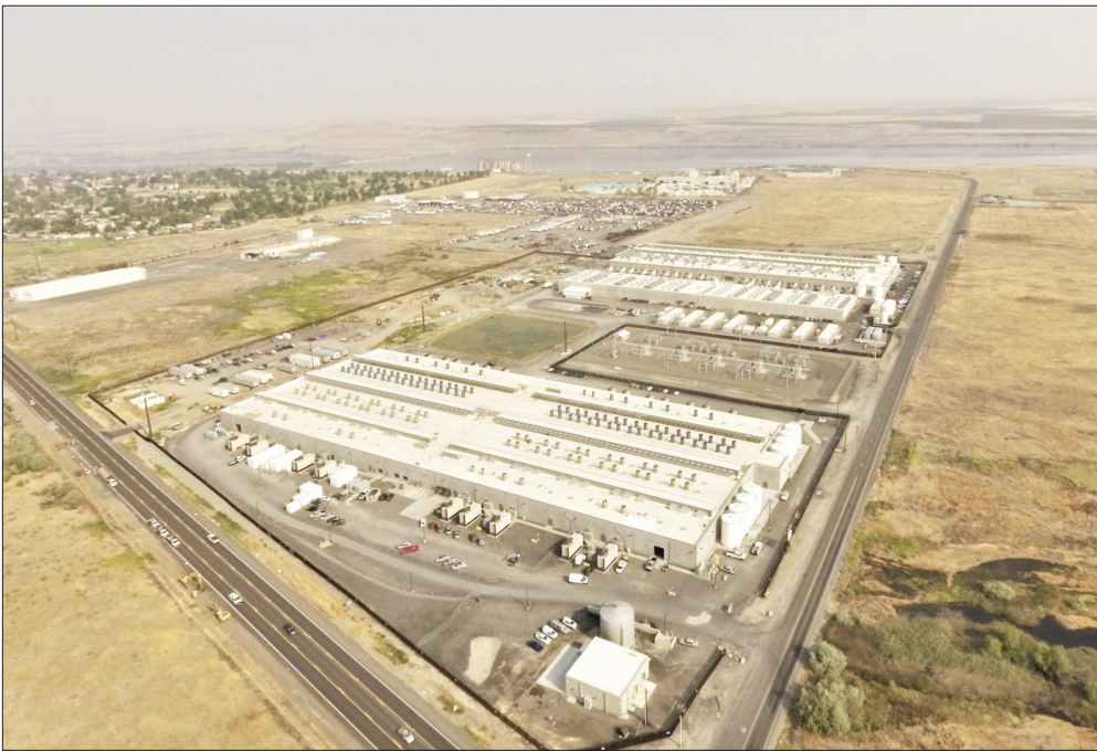
Photo contributed by James Thomas The Amazon data center in Umatilla is one of four sites in Umatilla and Morrow counties that have been completed since 2010, with at least two more on the way.
