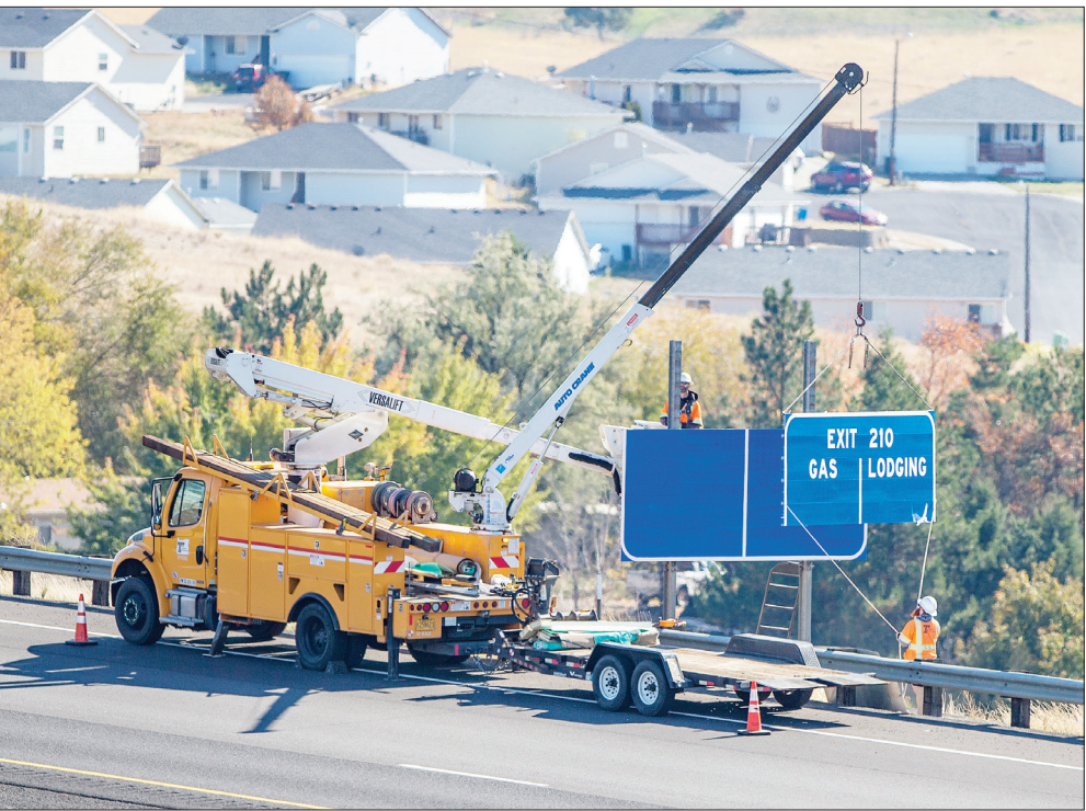
Staff photo by Ben Lonergan A pair of Oregon Department of Transportation workers raise a new interstate logo sign into place near Exit 210 on Interstate 84 westbound. For-profit businesses who wish to have their logo on a highway sign along I-84 between Hermiston and Pendleton pay $378 per sign, per year.
