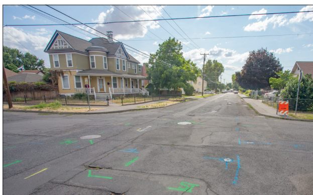
Staff photo by Ben Lonergan The intersection of Southeast Ninth Drive and Byers Avenue in Pendleton shows signs of wear with cracks and potholes. Byers Avenue is on the city's list of road repair projects.
