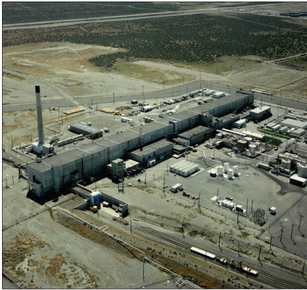
Contributed Photo, File A new federal report says that a massive building at the Hanford Nuclear Site is worse off than managers thought.
