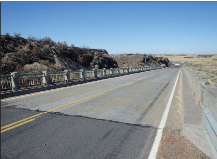
Photo contributed by the Oregon Department of Transportation The Oregon Department of Transportation in 2020 plans to shut down this 67-year-old railroad overpass bridge on Highway 37 in Umatilla County for five weeks while crews work on major repairs.
