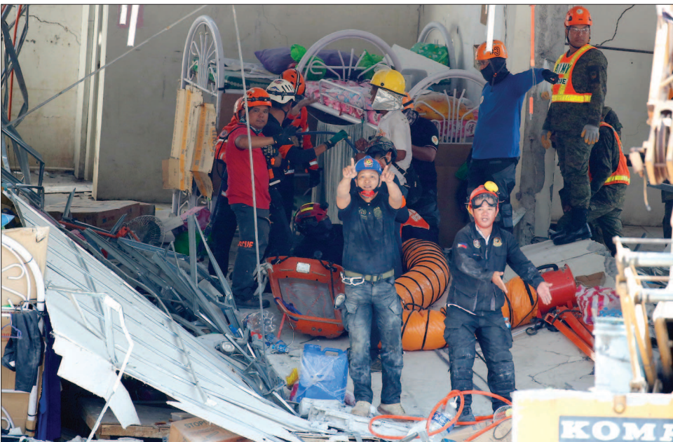
Rescuers gesture to clear the way following the discovery of another survivor in Monday's magnitude 6.1 earthquake that caused the collapse of a commercial building in Porac township, Pampanga province north of Manila, Philippines, on Tuesday. A strong earthquake struck the northern Philippines Monday, trapping some people in a collapsed building, damaged an airport terminal and knocked out power in at least one province, officials said.
