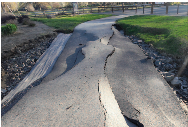
Staff photo by Jade McDowell A section of the Oxbow Trail leading into Riverfront Park in Hermiston has collapsed after being covered with flood waters for several days.
