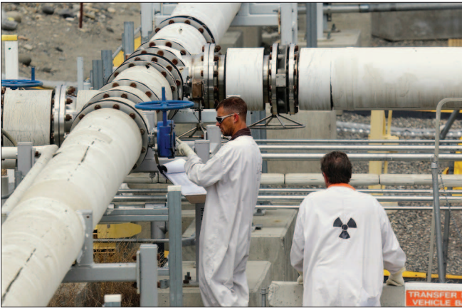
AP Photo/Ted S. Warren, File In this July 9, 2014, file photo, workers wearing protective clothing and footwear inspect a valve at the “C” tank farm on the Hanford Nuclear Reservation near Richland, Wash.
