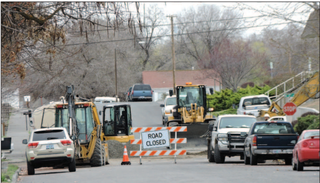
Staff photo by Jade McDowell Southeast Seventh Street is closed as crews work to install a new, larger sewer line to serve the south side of town.
