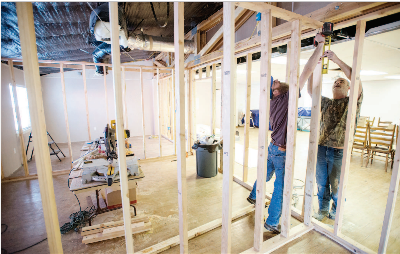
Richard Carnes, left, and Brad Cole put up a wall while building rooms for the new Eudora Wilson House elderly care facility in Pilot Rock.
