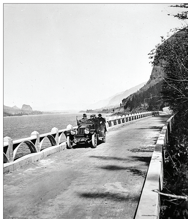
Courtesy of Historical Society Research Library/ A section of concrete road near Multnomah Falls, circa 1915. Featured in "Experience Oregon," a new permanent exhibit at the Oregon Historical Society.
