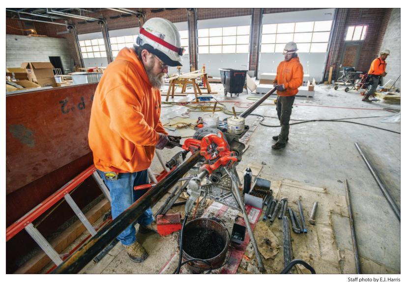
Workers cut a section of pipe for a sprinkler system while working on the building site for the new fire station on Wednesday in Pendleton.
