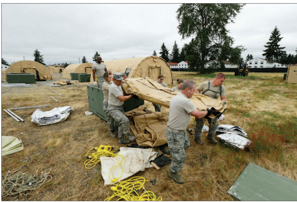
In this May 24, 2016, file photo, Washington Air National Guard soldiers from Fairchild Air Force Base in Spokane, Wash., work to assemble temporary living structures at Joint Base Lewis-McChord in Washington to train for emergency response in case of a natural disaster. A new state report says Bend would be the center of Oregon's emergency response in the worst-case scenario of a catastrophic earthquake along the Cascadia Subduction Zone off the Oregon Coast
