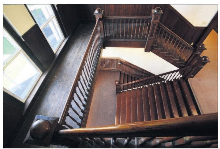
Restoration work has already begun on the main staircase to the third floor of the Milton-Freewater City Hall building where a layer of paint and been stripped and the wood is being refinished.
