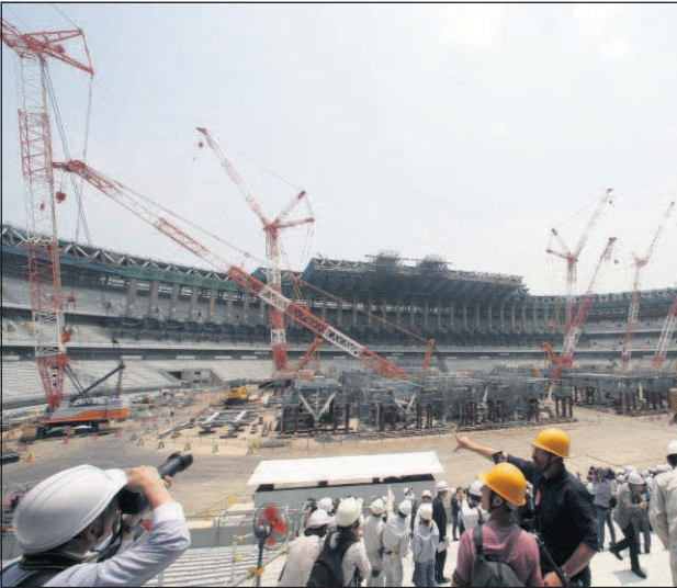
AP Photo/Koji Sasahara Journalists take photos of new National Stadium under construction during a media tour to the venue of the Tokyo 2020 Olympics in Tokyo.
