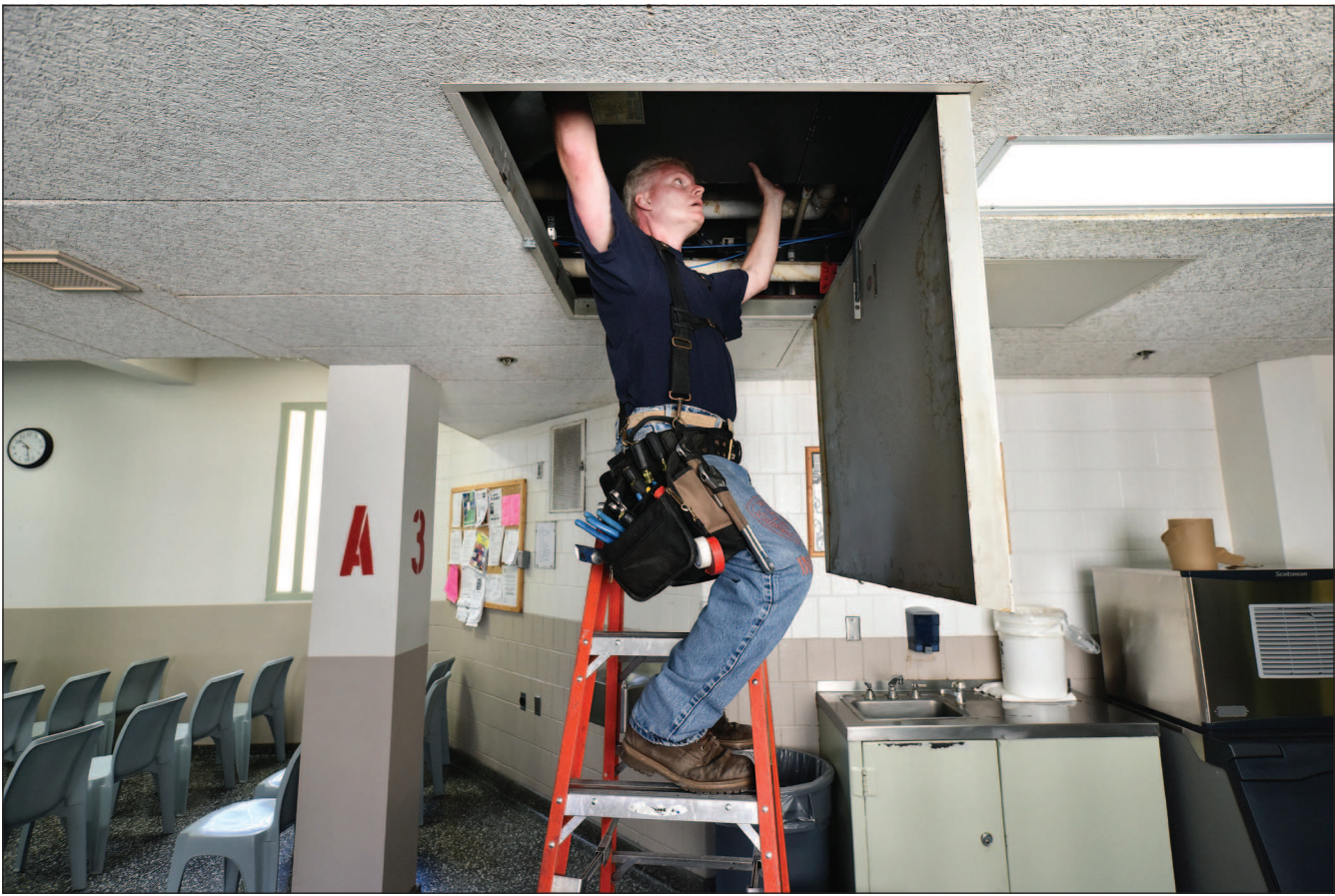
Above: Inmate Adam Anderson checks air-flow belt drives in the day room of one of the housing units at EOCL. He works in the HVAC department of the prison. Left: Anderson gets a pat-down before heading through a security checkpoint on his way to work at the prison physical plant. All 1,700 inmates are subject to random checks. Below: Anderson checks a Telmate kiosk to see if he has any emails in the commons area of his housing unit. He carries an MP3 player which can store photos and messages that have been approved by prison staff.
