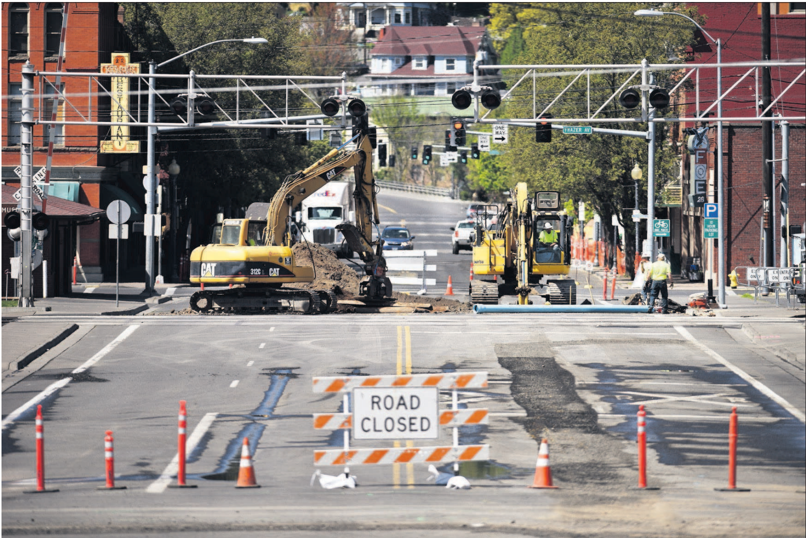
A pair of excavators work on replacing a water main near the intersection of Main Street and Frazier Avenue on Tuesday in Pendleton. Staff photo by E.J. Harris
